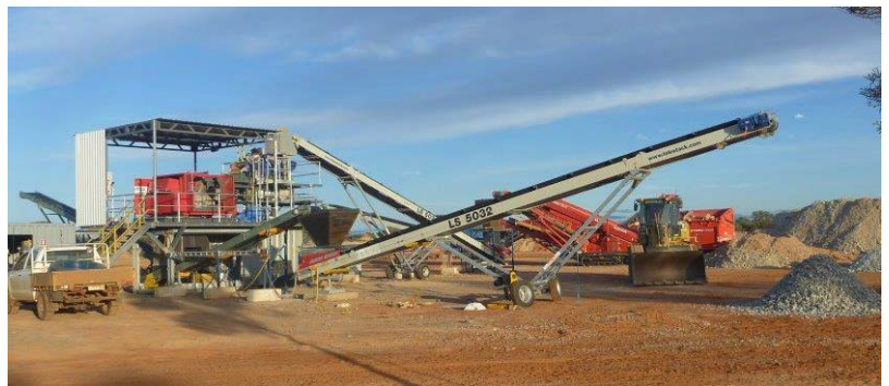
Figure 4: Sorting plant and Product slewing conveyor
