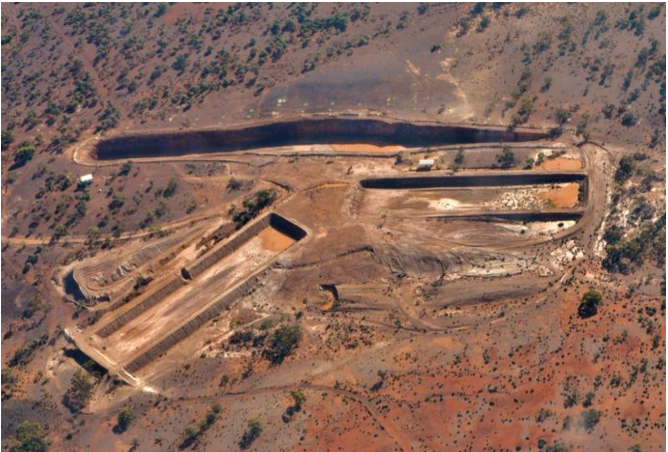
Zelica open pit showing constructed vat leach ponds and pre-stripped open pit
